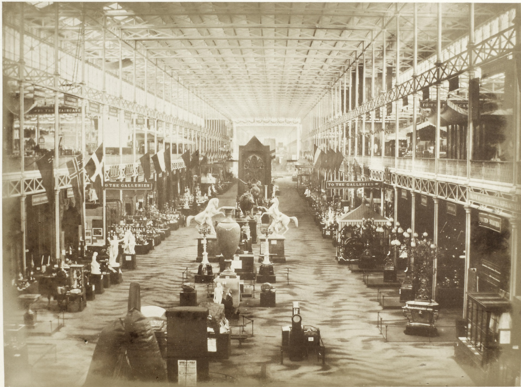
VIEW OF EASTERN NAVE.
